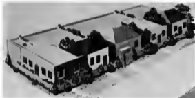
Figure 64. Depot warehouses, power houses, and similar large structures in urban areas are often made to appear to be a group of smaller buildings characteristic of the locale. Roof lines are varied with wooden framework covered with burlap or fine mesh wire netting to simulate sloping hip roofs. If pavement presents planting real shrubbery, two or three dimensional false shrubs of steel wool or glass fiber will disrupt the shadows. Firewalls projecting above a roof can be transformed into garden walls or hedgerows on simulated property lines. Monitors, elevator shafts, and other projections can be disguised as small buildings.
